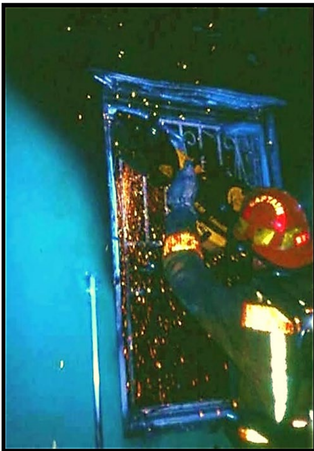
CAPTAIN BILL GUSTIN WORKING ON SOFTENING UP THE STRUCTURE AS HE CUTS BARS OFF A WINDOW
